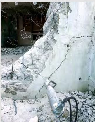
Demolition of concrete and reinforced concrete
