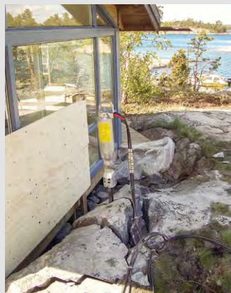
Demolition of rock and natural stone
